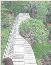
Tree House, Jubilee Street, Stepney [6a Architects]
