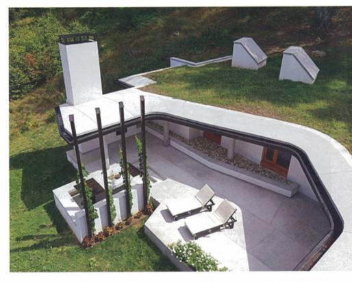
PIR on top, and then 120mm of soil planted with grass on top of that.
